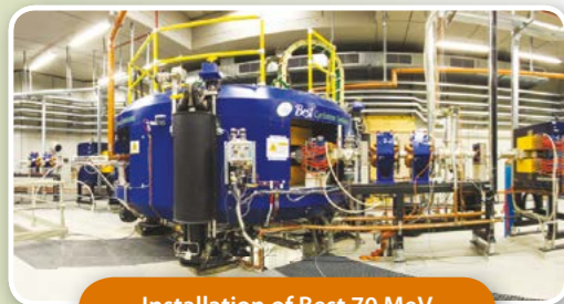
Installation of Best 70 MeV Cyclotron at INFN, Legnaro, Italy
