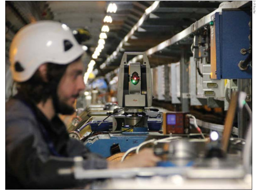
Fieldwork Alban Vieille of the accelerators, survey and geodesy section aligning a LHC collimator.
