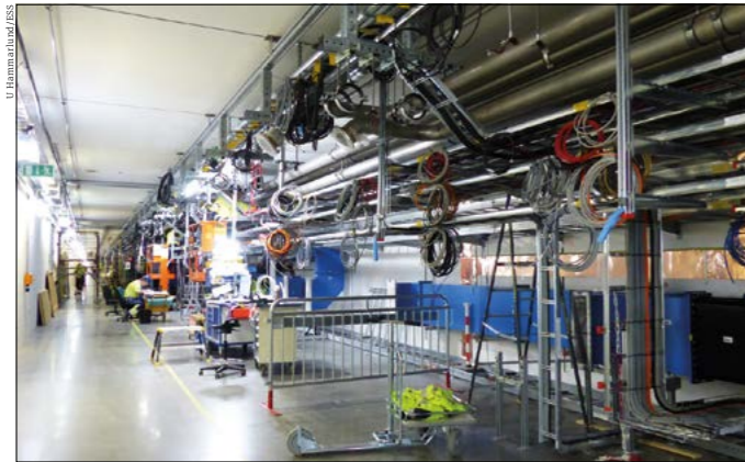
Cabling Installation of part of the 5 MW proton linac.
