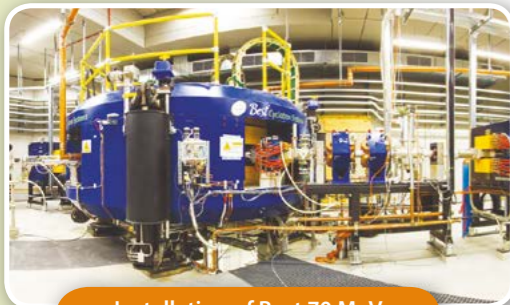
Installation of Best 70 MeV Cyclotron at INFN, Legnaro, Italy
