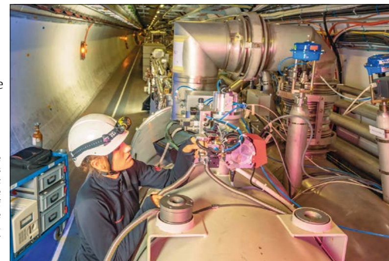
Engineering prowess Natalia Magdalena Koziol, an engineer from Poland, is responsible for quality assurance of the LHC's insulation vacuum during Long Shutdown 2.
