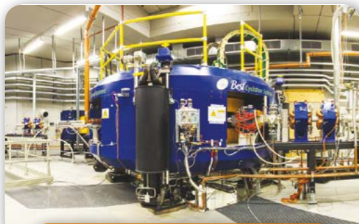
Installation of Best 70 MeV Cyclotron at INFN, Legnaro, Italy
