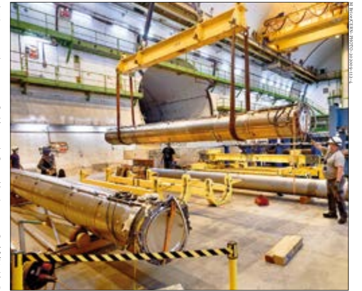
Dump upgrades Upgraded LHC external dumps with new instrumentation, beam windows and support systems being fitted into their new frames, ready for installation.
