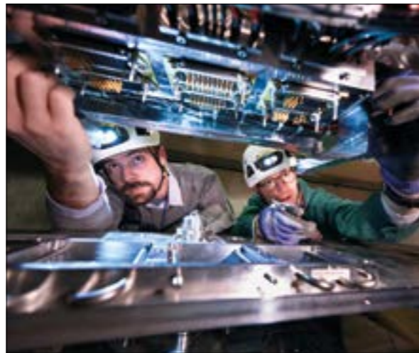
New collimators Left: new dispersion-suppressor collimators being installed near ALICE in 2020, where they will clean beam losses at the HL-LHC. Right: checks during collimator installation in one of the SPS-to-LHC transfer lines in November 2019, as part of the LHC Injector Upgrade Project.
