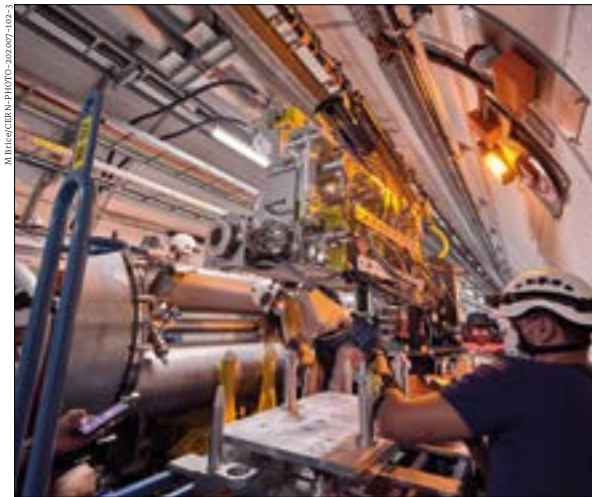
New collimators Left: new dispersion-suppressor collimators being installed near ALICE in 2020, where they will clean beam losses at the HL-LHC. Right: checks during collimator installation in one of the SPS-to-LHC transfer lines in November 2019, as part of the LHC Injector Upgrade Project.
