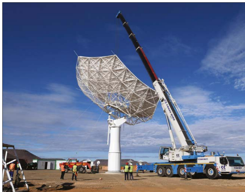
Rising up "SKA-MPI", the Max Planck Society-funded prototype dish, being assembled at the South African site in early 2019.
