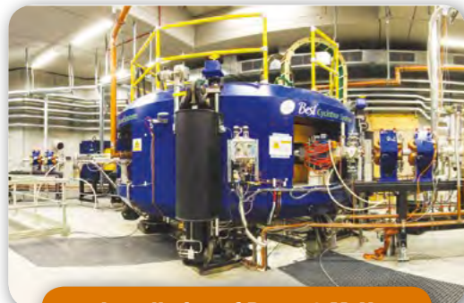
Installation of Best 70 MeV Cyclotron at INFN, Legnaro, Italy
