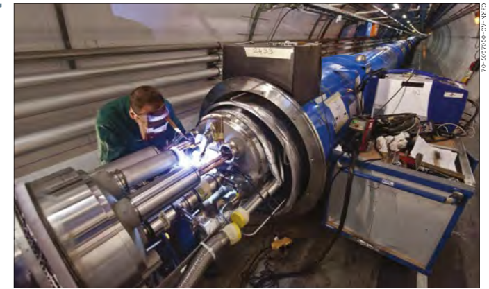
Downtime Welding a dipole-magnet interconnect in sector 3-4 in April 2009.
