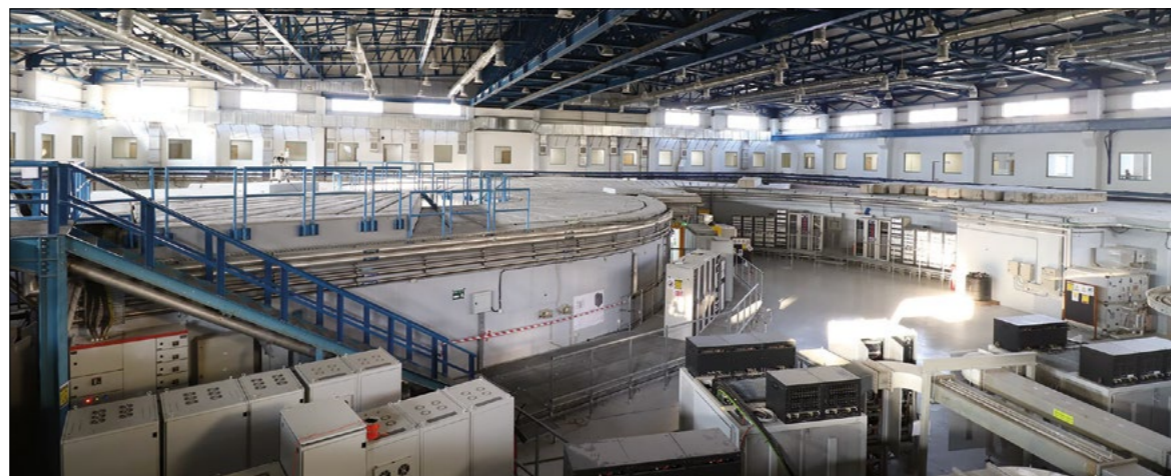
Illuminating The SESAME booster (inner ring) and storage ring, concealed behind their concrete shielding.
