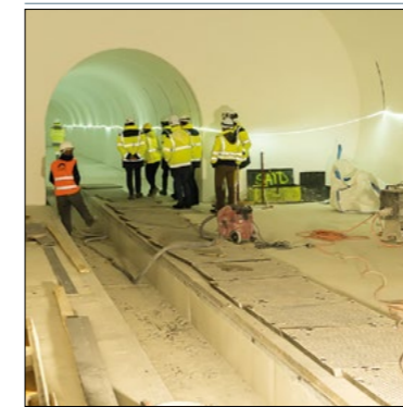
Closing in Civil engineering for the High-Luminosity LHC completed. 7
