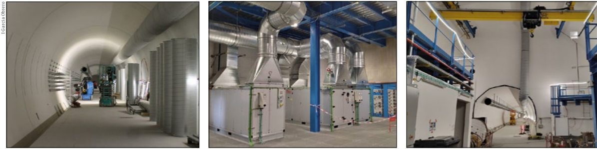
Buildings and infrastructure The new gallery at Point 1 (ATLAS) for power converters and other equipment (left); the surface building for cooling and ventilation at Point 5 (CMS) (middle); and the underground service cavern (right).
