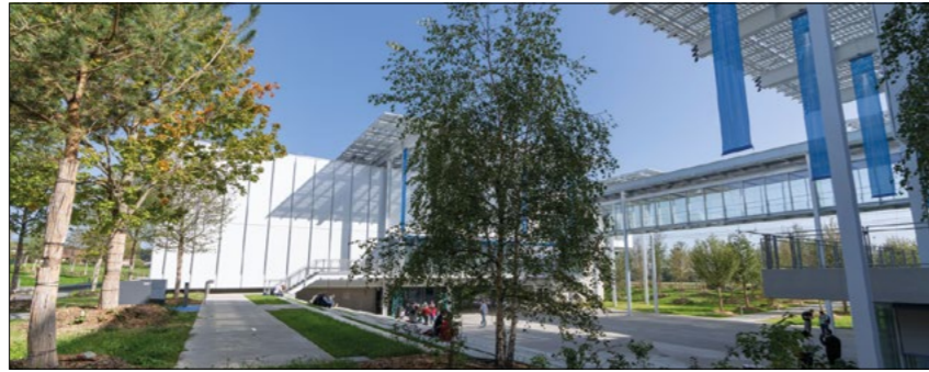
Efficient CERN Science Gateway is fitted with almost 4000 m 2 of solar panels that also provide energy for other CERN buildings.
