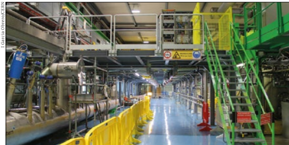
Inner-triplet string Top: the key elements constituting the new insertion regions for the high-luminosity LHC experiment, showing the quadrupole (Q) and dipole (D) assemblies, superconducting-link feedboxes (DFHX and DFH), cryogenic distribution line (SQXL) and auxiliary equipment. Above: the string in SM18 (left) and the installation of electrical infrastructure and signal cables in December 2023 (right).
