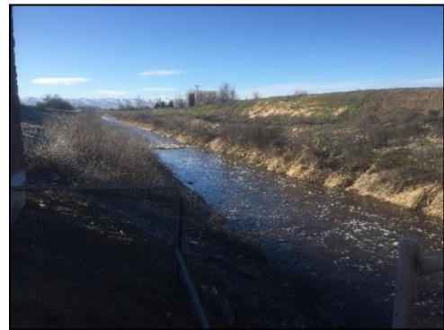
Figure 47 – Sulphur Creek Wasteway downstream view
