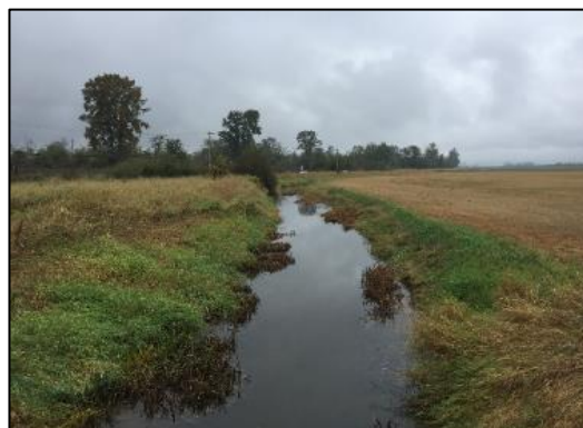
Figure 11 – Lower Big Ditch upstream view
