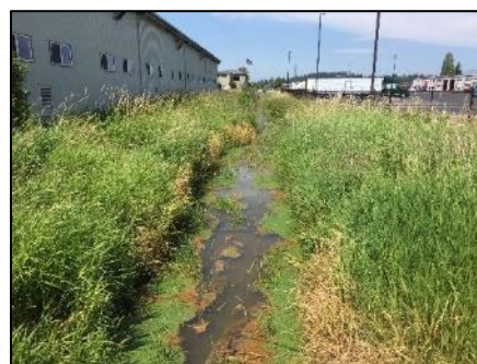
Figure 8 – Upper Big Ditch upstream view
