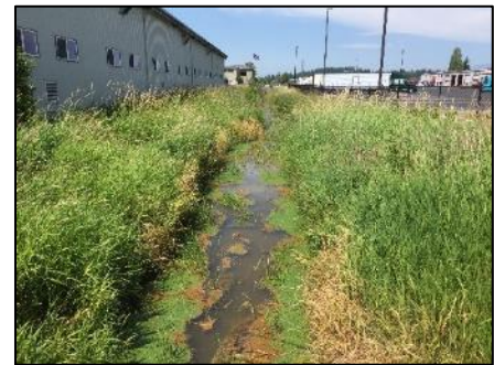
Figure 8 – Upper Big Ditch upstream view
