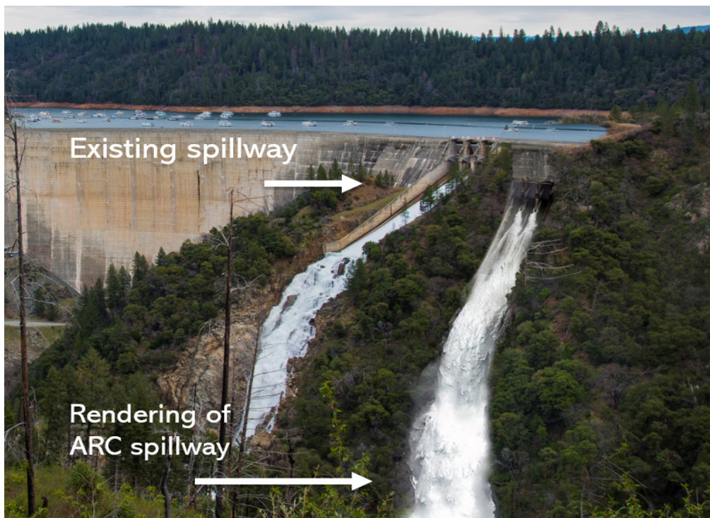
Figure 2-4. The ARC Spillway will have the capacity to pass the flood of record (~50,000 cfs) without use of the primary spillway. Credit: Yuba Water Agency.
