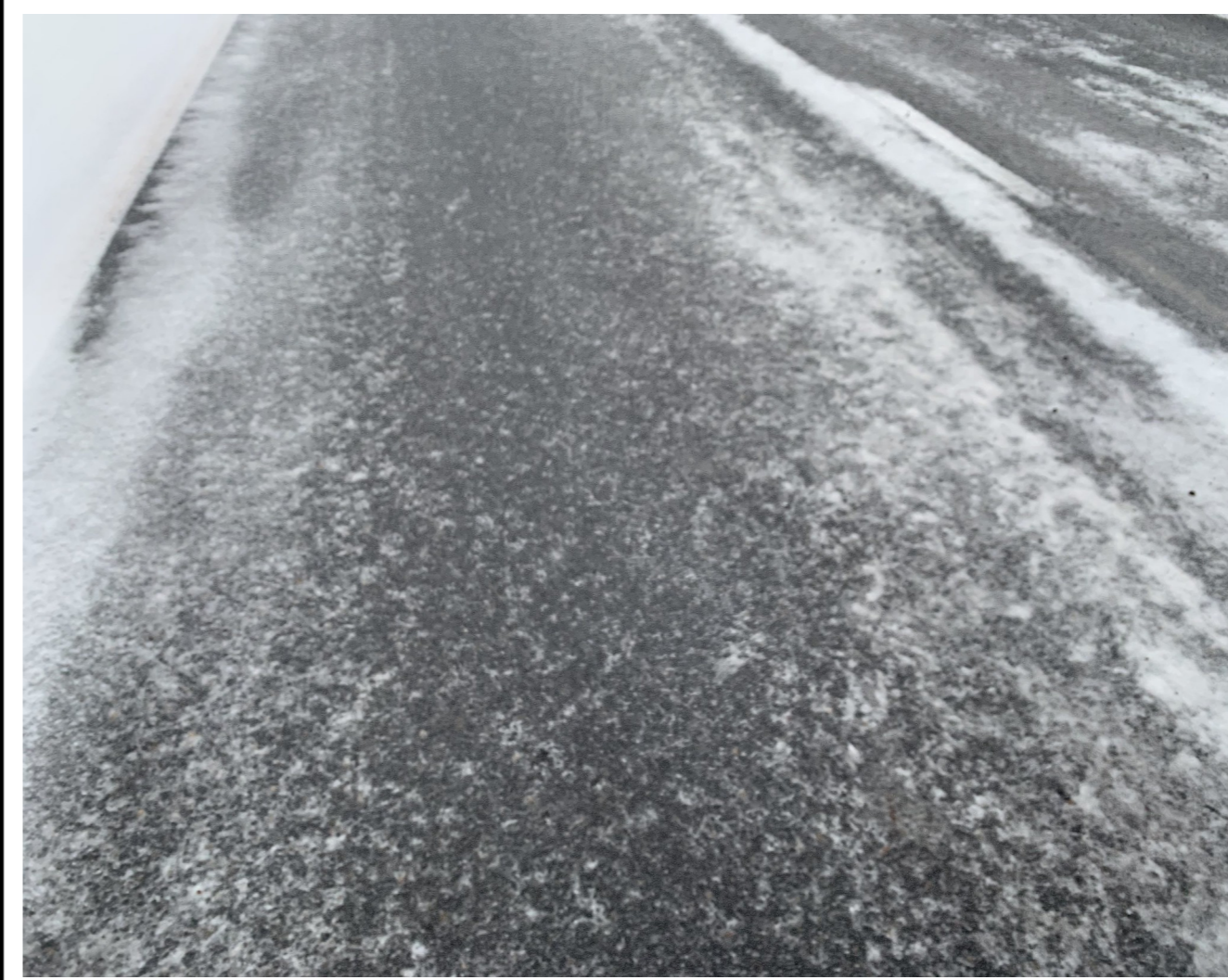
Thick Sheet of Ice Covering I-84 in the Columbia River Gorge in OR (courtesy: Oregon Department of Transportation)
