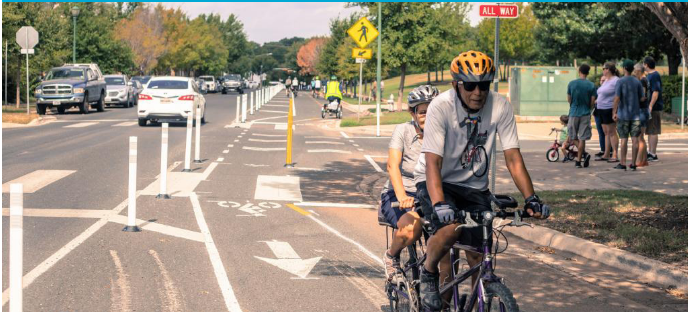
Figure 13: Separated bicycle lane in Austin, Texas, USA with increased ridership. Source: City of Austin
