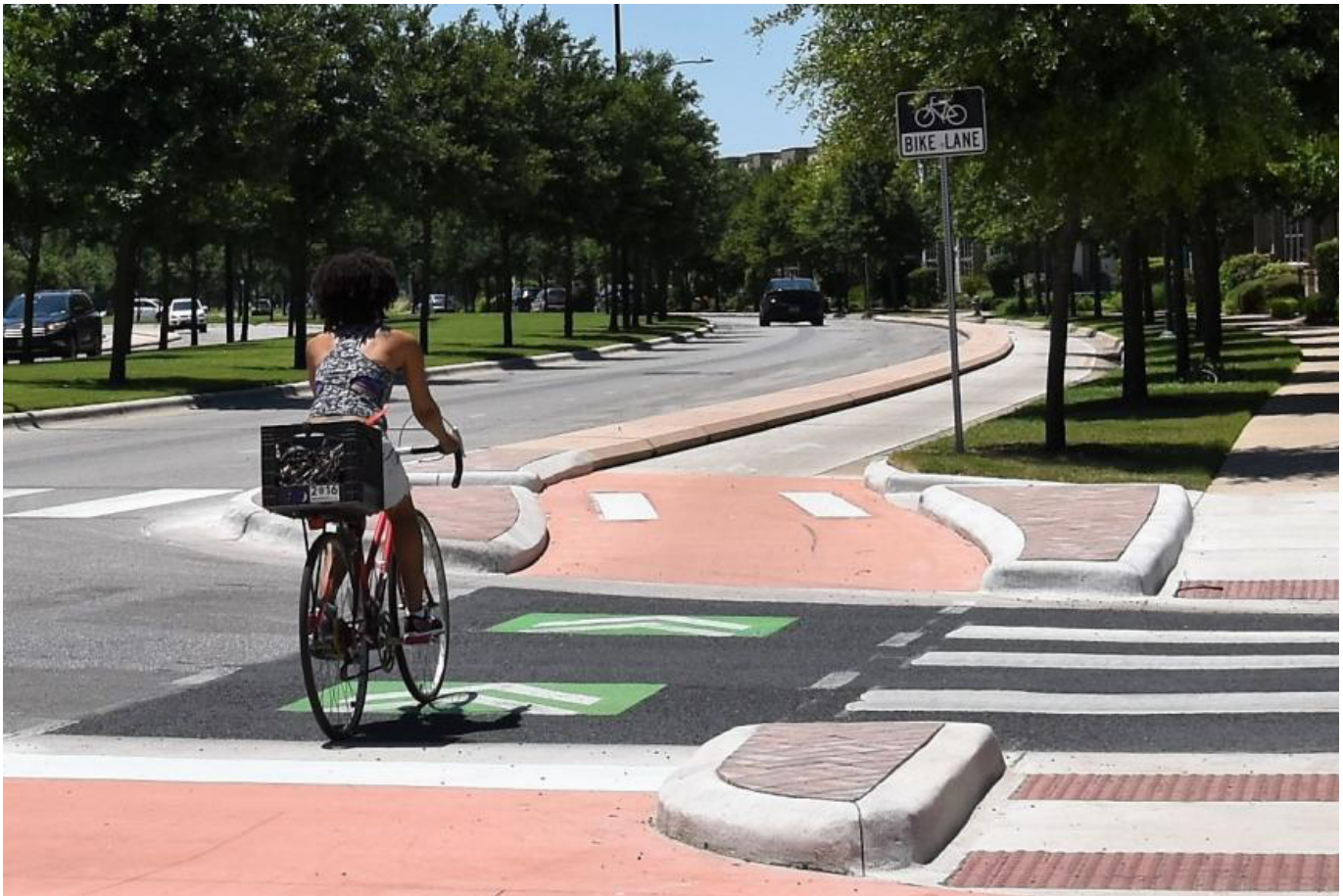
A separated bike lane using a concrete curb in Austin, TX, USA that considers context in selection of facility type. Source: City of Austin .
