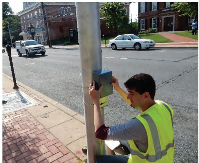
Pyro box installation
