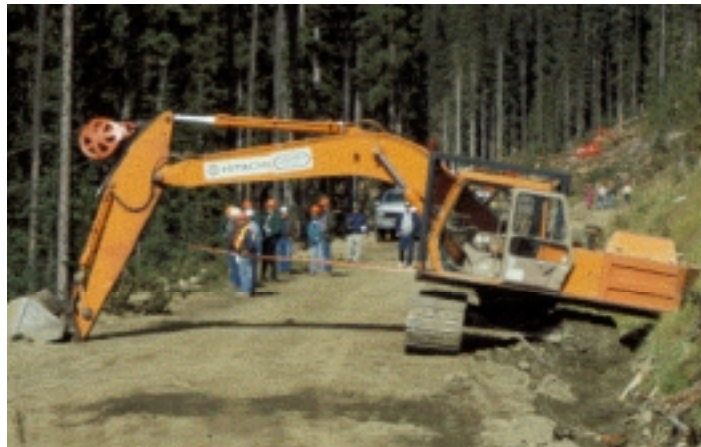
Figure 5: Excavator used as mobile tailhold
