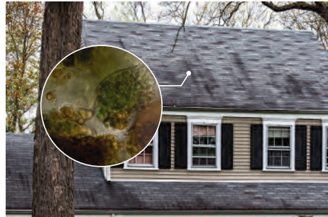
Gloeocapsa magma is blue-green in color, but surrounds itself with a dark brownish-black shell to protect against the sun's rays. The dark shell causes the telltale streaking on the roof.
