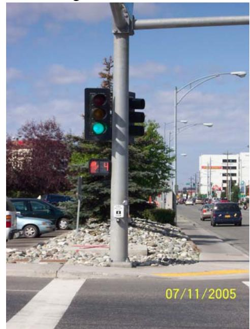
Install “PORK CHOP” islands between the right turn and thru lanes at large intersections with high right turning movement to help get pedestrians and bicyclists beyond the right turning vehicles and onto a raised island where they can then cross the thru traffic stream during a WALK interval.
