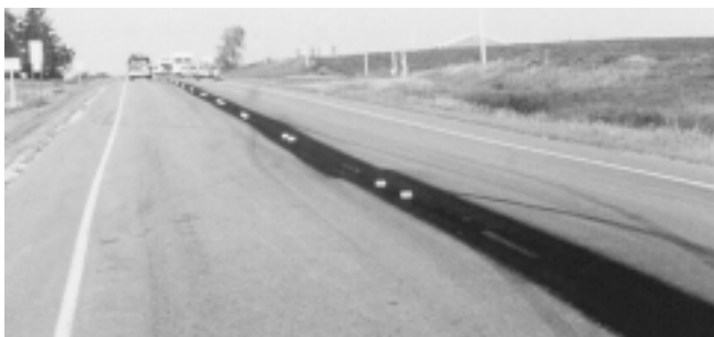
Figure 8.3. Fog seal on centerline before seal coat to prevent excess absorption
