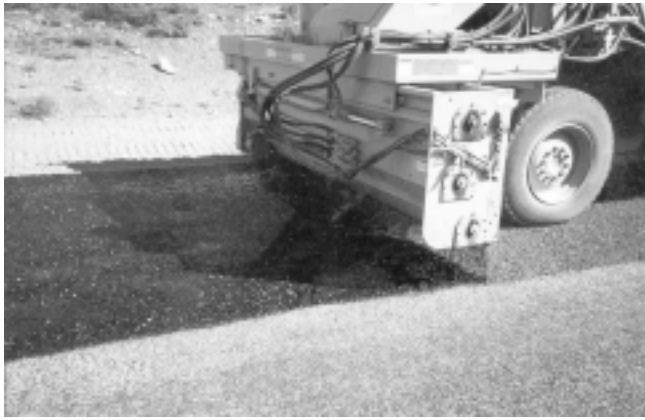
Figure 7.21. Cover aggregate spreader in action
