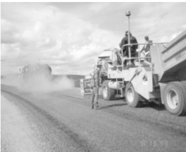
Figure 7.19. Applying second layer of aggregate
