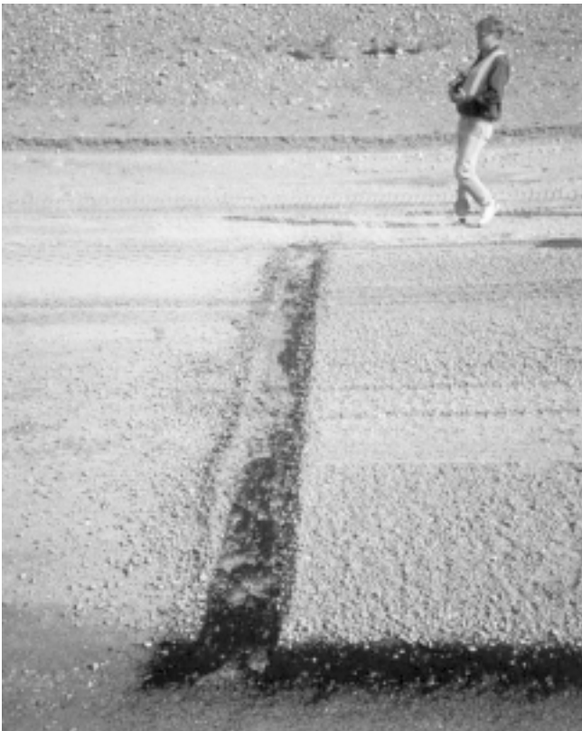
Figure 7.15. Cleaning for transverse joint area
