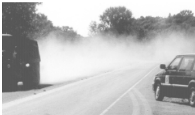
Figure 8.4. Evidence of dusty aggregate
