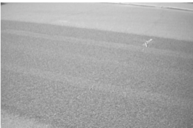
Figure 7.3. The rubber mats are covered with aggregate from the aggregate spreader.
