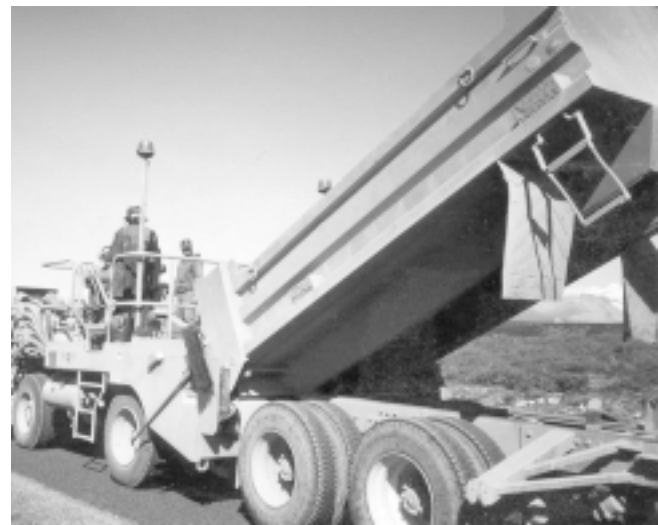
Figure 7.20. Loading aggregate spreader
