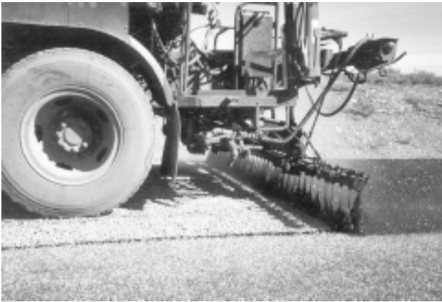
Figure 7.18. Emulsified asphalt distributor in action
