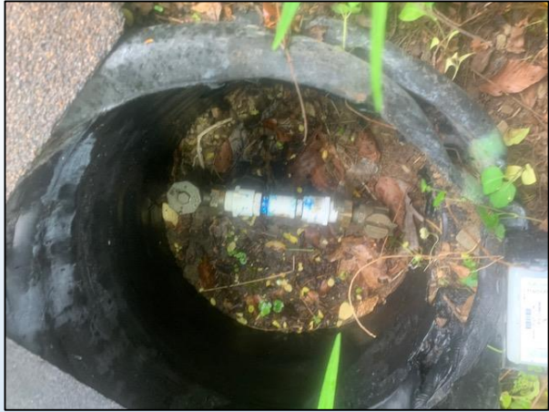
Jumper installed after meter was removed
