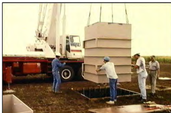
Installation of Large Precision-Weighting Lysimeter
