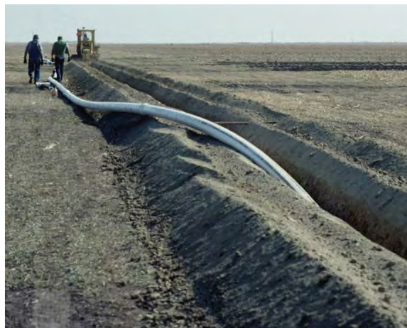
Figure 9.11. Installation of a buried pipeline for irrigation water delivery.
