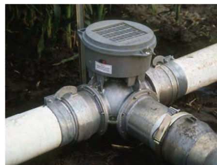
Figure 10.19. Tee-type surge irrigation valve.
