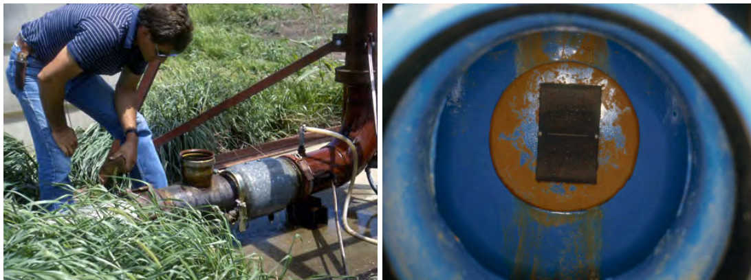
Figure 15.7. Inspection for check valve leakage in CCVA.
