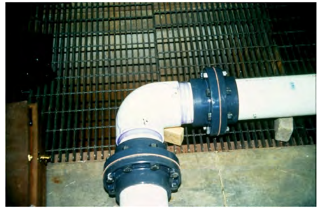
Profile disturbed by elbow
