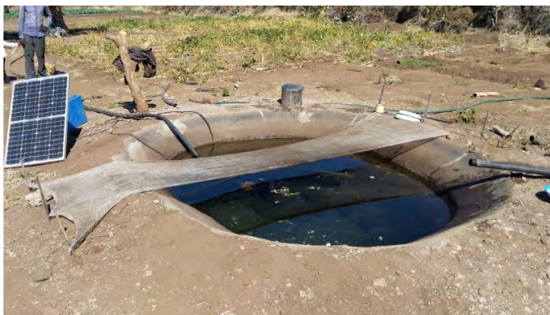
Figure 9.5. Water delivery system for groundwater from the shallow alluvial aquifer of the Shashe River, Zimbabwe. A solar pump is used to deliver water from the concrete-lined storage pond to a nearby field, and the net provides shade for fish. (Photo courtesy of Annelieke Duker, IHE Delft Institute for Water Education.)
