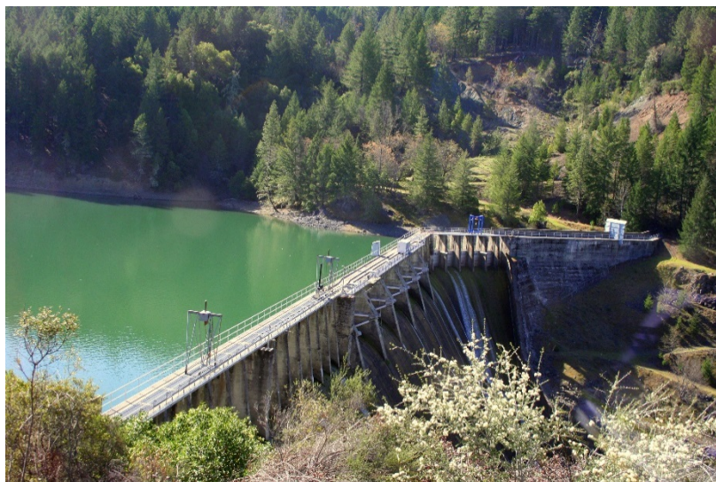
Figure 2.4. Photo of Scott Dam on the South Fork Eel River. Source: Sonoma County Water Agency.
