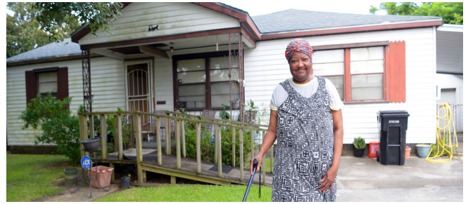
Betty Kennedy, recipient of DRA funding to replace damaged roof in New Orleans, LA.
