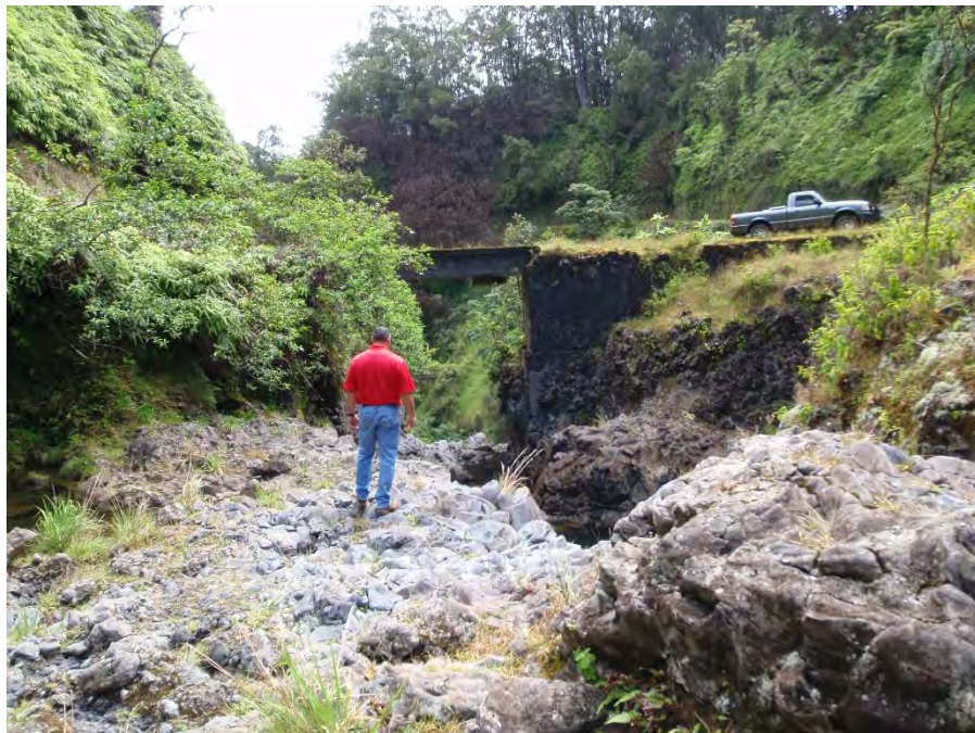
Downstream view of bridge from the dam wall
