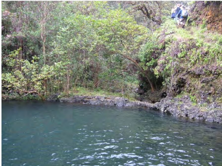
Dam wall in plunge pool downstream view
