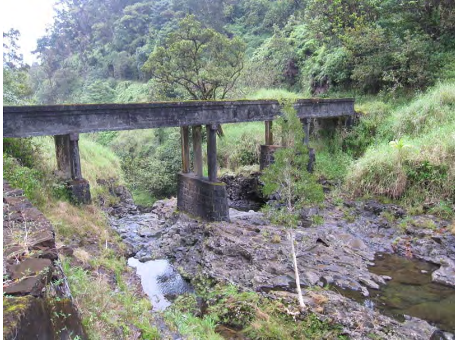
Downstream view of bridge from diversion
