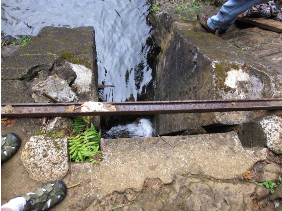
On top of diversion intake tunnel
