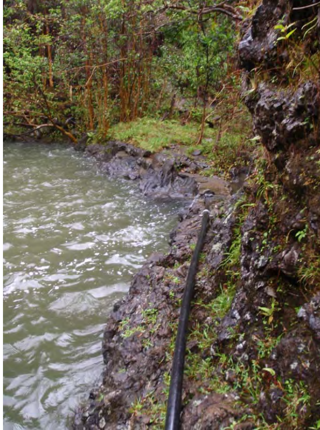
Pipe to dam (gh002d-017p-041012)
