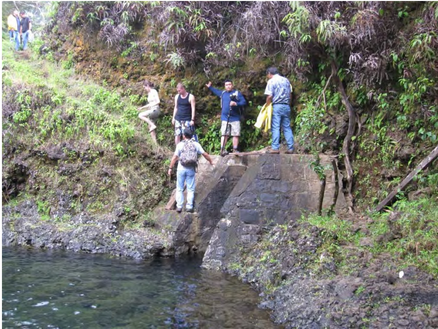
Diversion intake to left of waterfall
