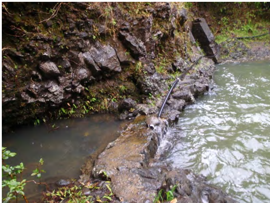
Dam wall with stream channel left and waterfall plunge pool right (gh002d-009p-041012)
