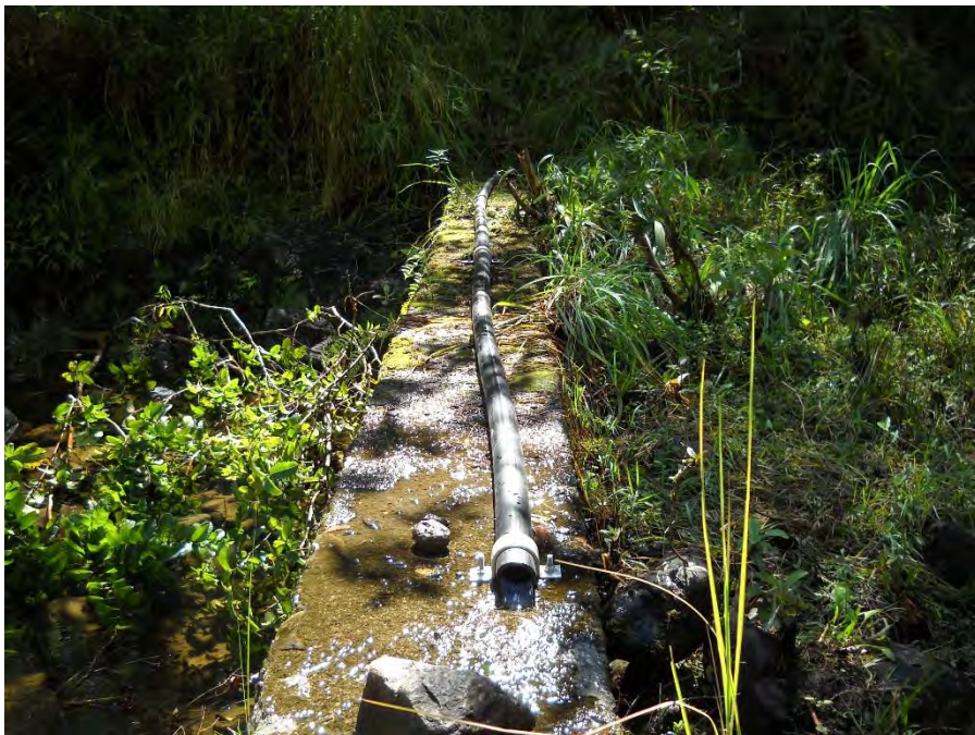
Pipe transferring water on diversion wall
