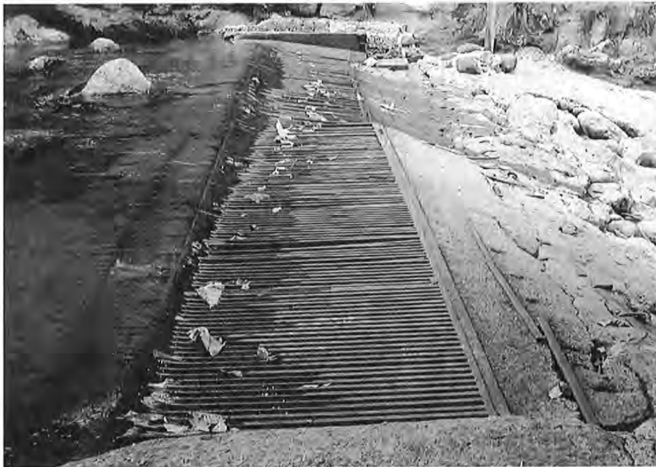
Figure 10. 'Īao Stream Diversion (below USGS Stream Gauge No. 16604500). Most stream flow is diverted into irrigation ditches.
