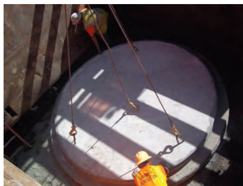
A crew installs a stormwater runoff system in downtown Seattle.
