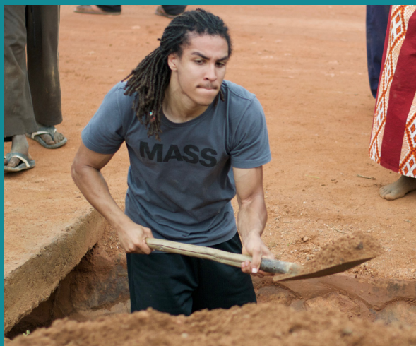
Josh on site at a construction project in Bugusera, Rwanda
