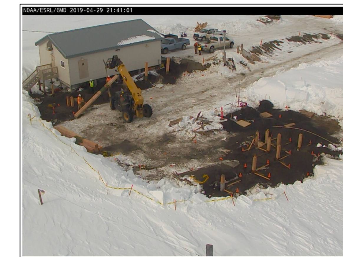
Piling foundation installation 29 April 2019
