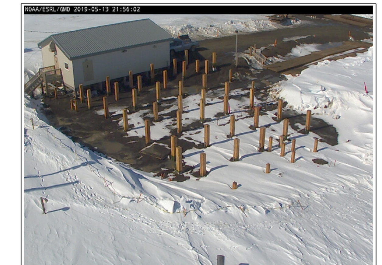
Piling foundation completed 13 May 2019
