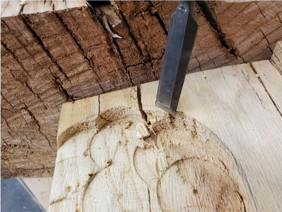
Figure 3. Final wood shaping with hand tools (chisels and hand sanding) to accommodate alarm bells.
