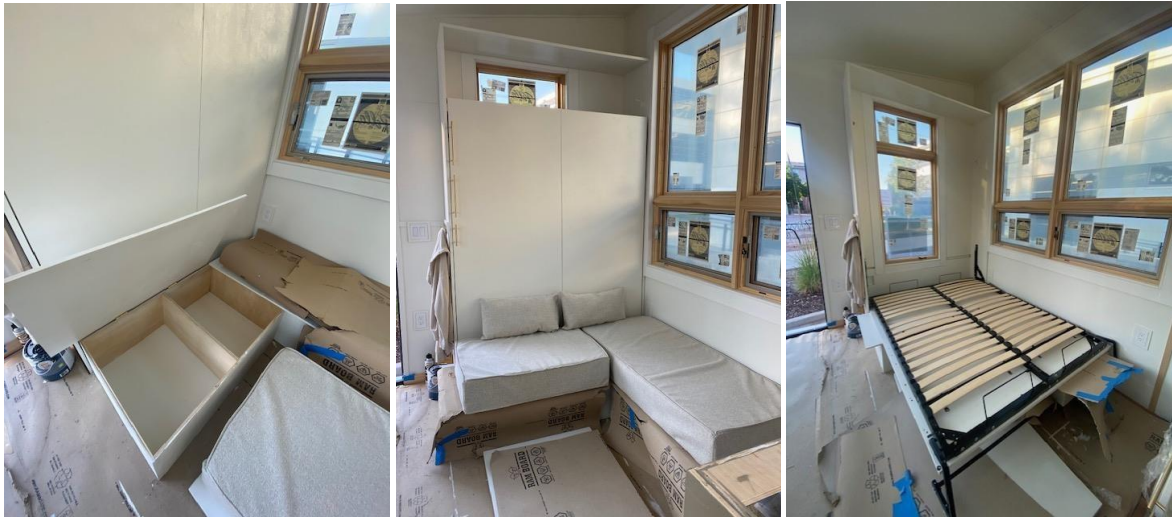
Image 12-13: Student kitchen countertop/workspace system pre-final product.*
