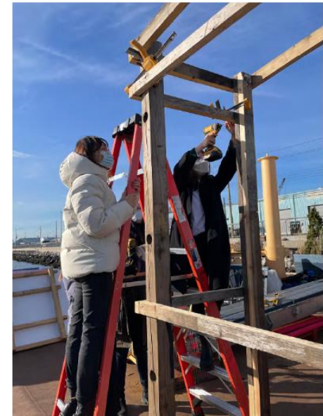
Construction on the barge
