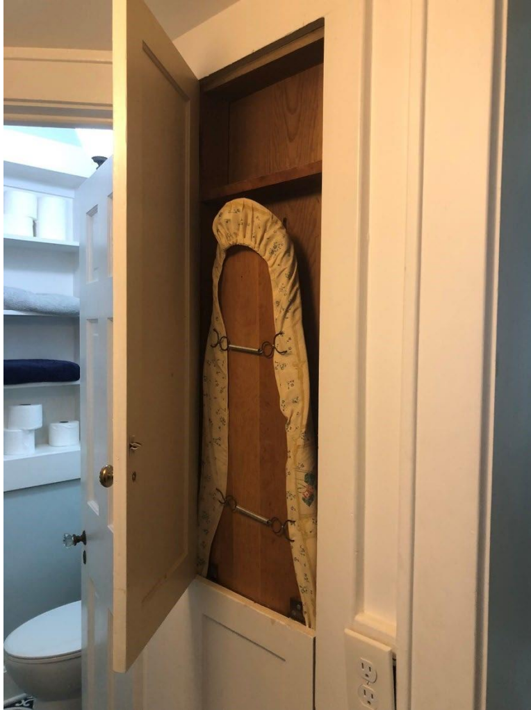
Figure 2. Ironing board cabinet from a house built in 1939. Photograph provided by the author, 2023.
