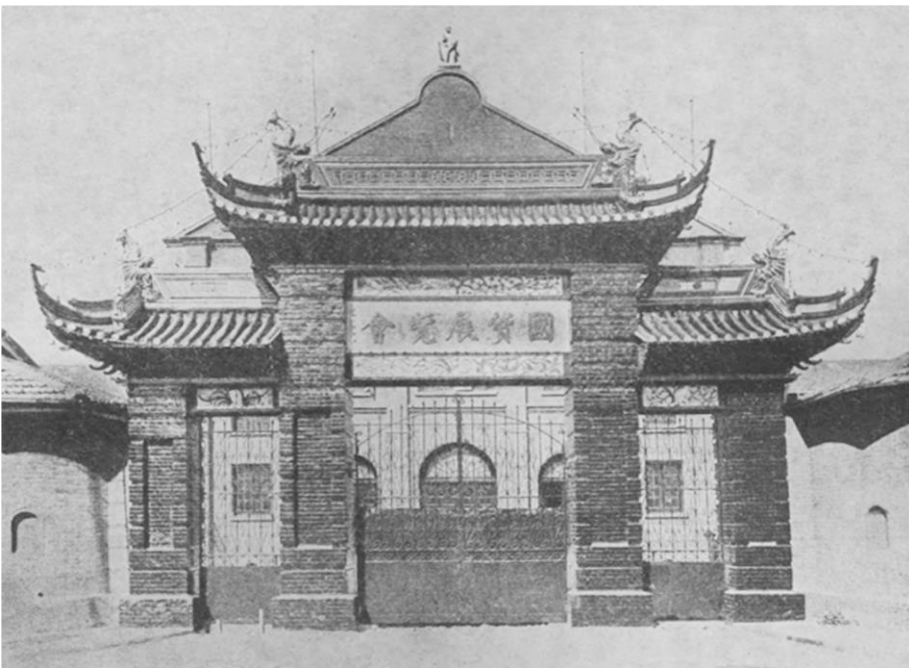
Figure 4. Front entrance of the National Goods Exhibition shows traditional Chinese characteristics: symmetrical front façade with three bays, upturned eaves, intricate carvings, and a plaque with calligraphy characters stating, “National Goods Exhibition.” Kai Wang, “Opening of the National Exhibition: Shanghai government showroom attached to the National Exhibition site” (Guohuo Zhanlanhui Kaimu: Guozhan Huichang Nei Fushe Chenlieshi Zhi Neiwaiguan,) The Young Companion (Liangyou) , November 1928, 12.
