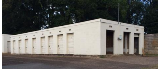
Proposed site of facility / Storage Building
