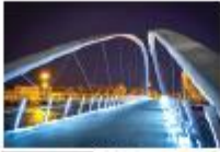
BRIDGE SEPTEMBER 2012 - OCTOBER 2014 CONNECTS [REDACTED]
