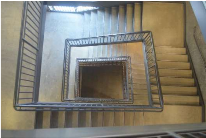
Figure 1. Site location A: 50-foot high, multi-level stairwell. All Hard surfaces with very little diffusion. This was the most reverberant space.
