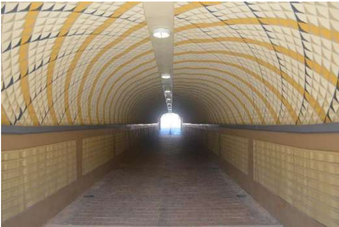
Figure 2. Site location B: 170-foot long pedestrian tunnel. Hard surface treatments create a semi-reverberant and highly diffuse environment.
