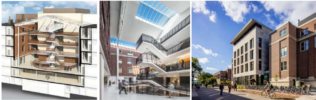
Figure 1: Left: Section of the courtyard and classroom addition looking east, center: atrium, right: east façade.
