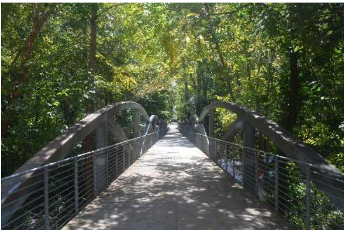
Figure 3. Site location C: 160-foot long pedestrian bridge. The lack of enclosure and reflecting surfaces makes this the least reverberant of the spaces.
