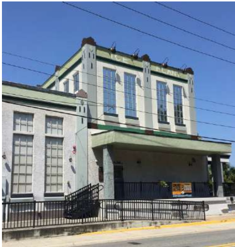
Figure 1. Exterior of Ice Plant building. September 8, 2019. (photo by author)
