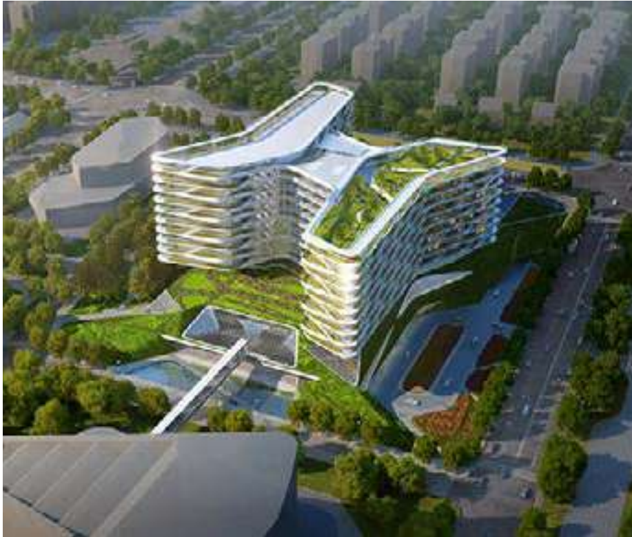
HOK Shanghai International Hospital Shanghai
