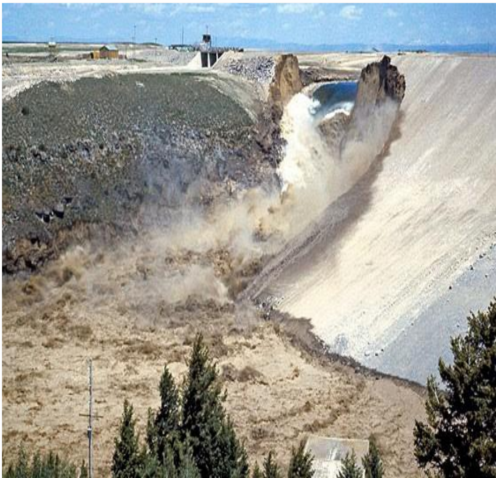
Figure 3.15.F. Teton Dam Failure, June 1976
