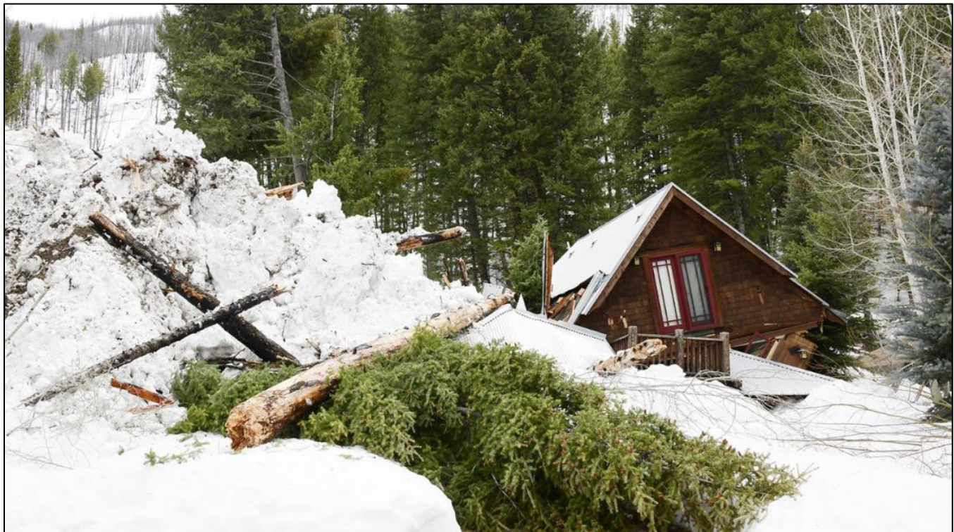
Figure 5-3. Home Near Ketchum Destroyed by an Avalanche in April 2019
