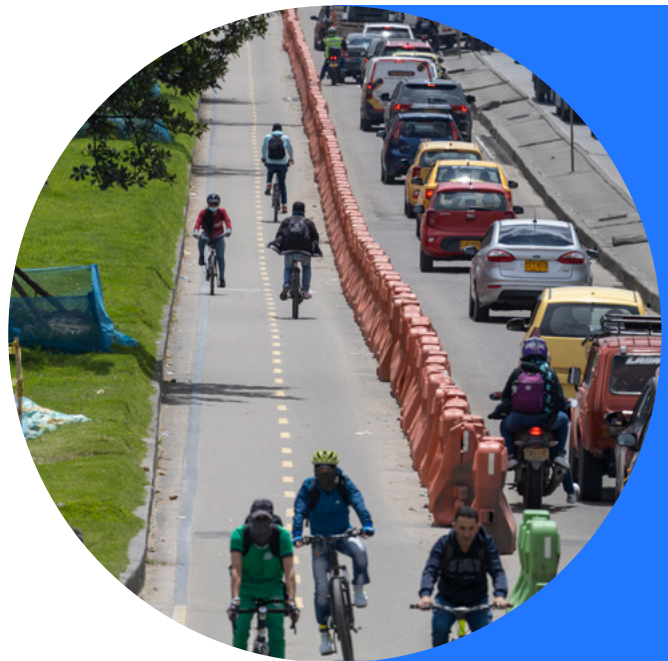
A two way bicycle lane in Colombia separated by temporary barriers. Source: Despacio
