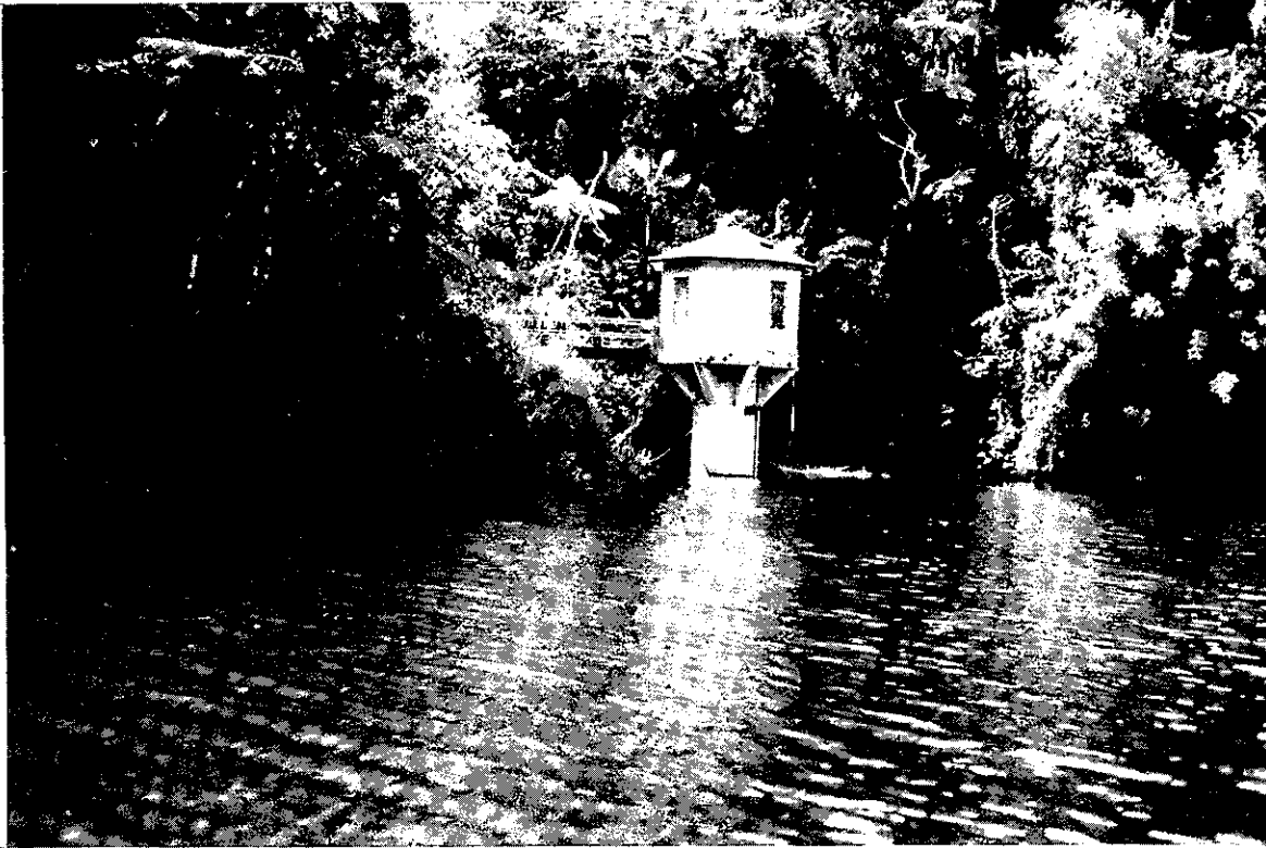
Figure 33. Outlet gate from Lake Garzas diverting flow to turbines and irrigation system on south coast.
