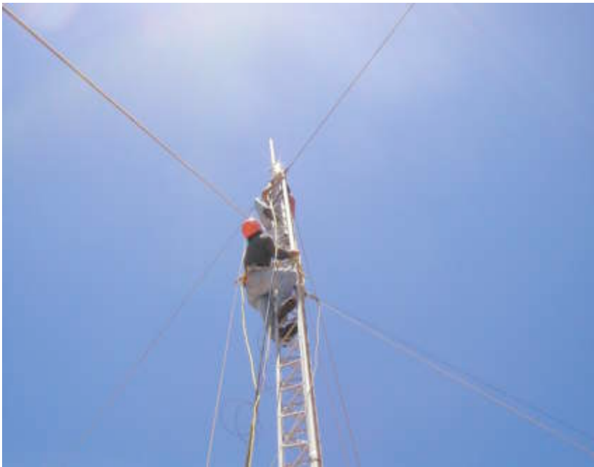
Figure 7.2: A climbable guyed tower.
