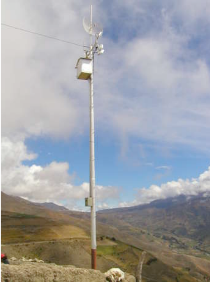
Figure 7.3: A simple self-supporting tower.
