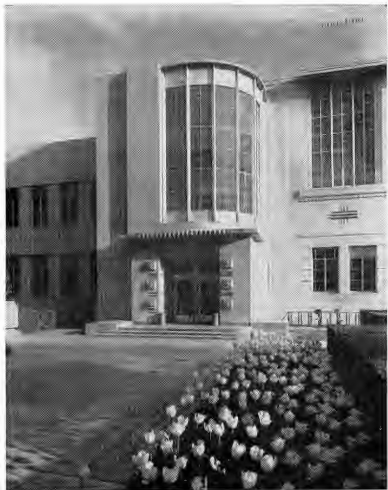
Entrance to administrative section of Library-Administration Building
