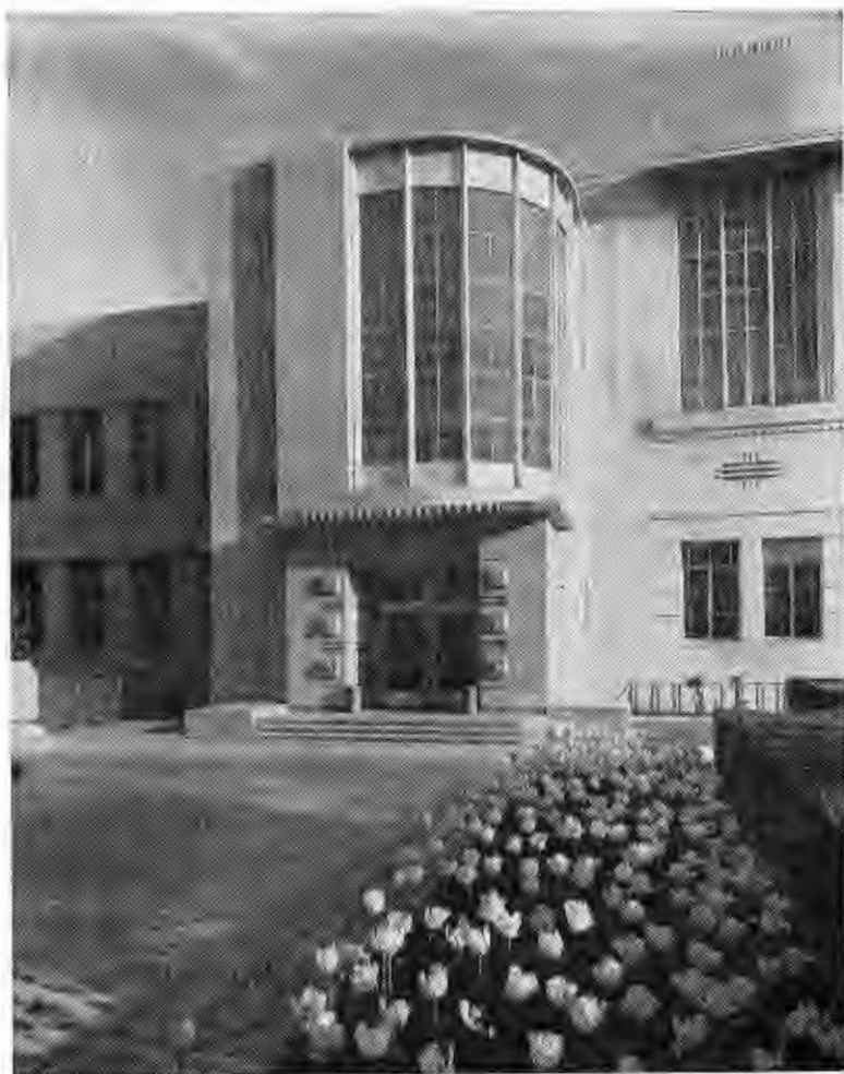
Entrance to administrative section of Library-Administration Building
