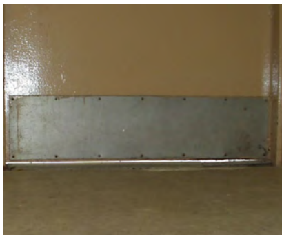
To check doors for possible rodent entry points, stand in the dark and look at the closed door with bright light shining behind it. (Photo L. Pinto)
