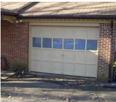
An attached garage is often the first stop for mice moving into residential homes. (Photo L. Pinto)
