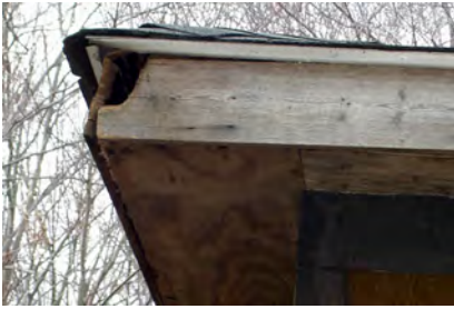
Seal, screen, repair or otherwise rodent-proof openings on and around the roof that can let rodents into the building. (Photo L. Pinto)
