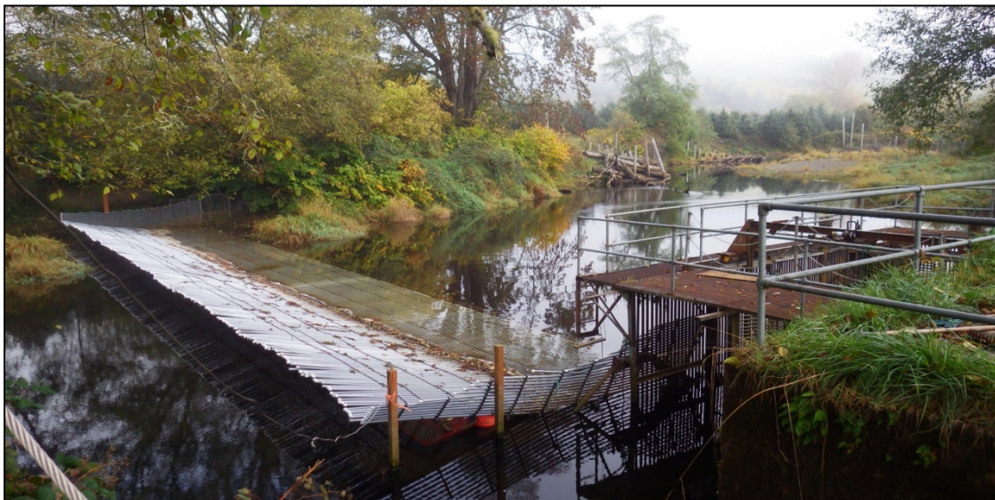
Figure 5.1.2: Lower Elochoman River adult weir configuration in 2016, located near the Foster Road Bridge. (Source: Patrick Hulett, WDFW.)
