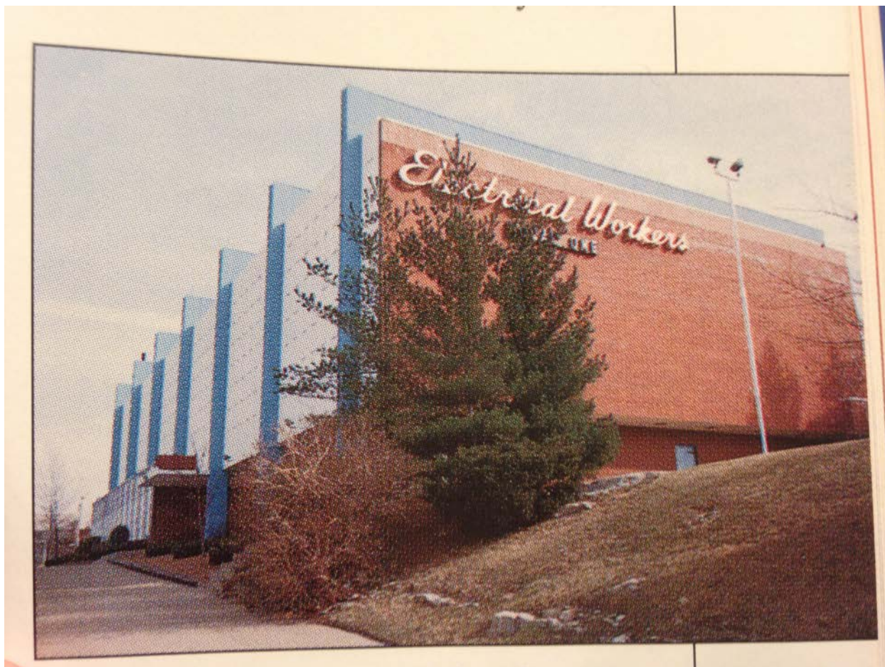
Figure 5: IBEW Building c. 1960, Electrical Worker's Journal
