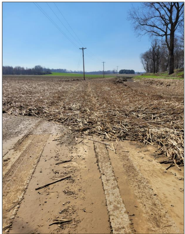
Road closed because road and ditch are now corn stalks for around ¼ mile. Nearest station showed a 3.8" rain event over two days. -Hans Schmitz (Purdue)
