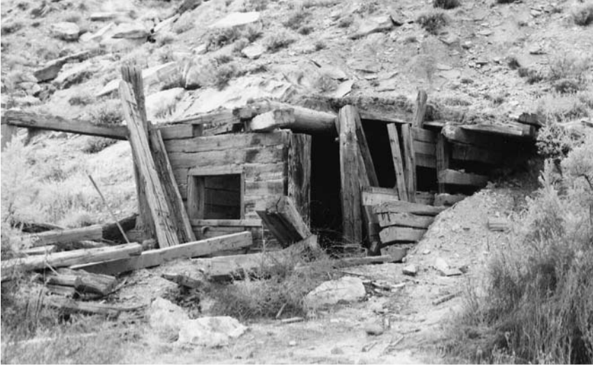
This structure built in the side of the hill near the mouth of Bitter Creek was Ed Herbert's garage according to John L. Malin. Photo from Wilford Hill files courtesy of Elsa Spaulding Hill.
