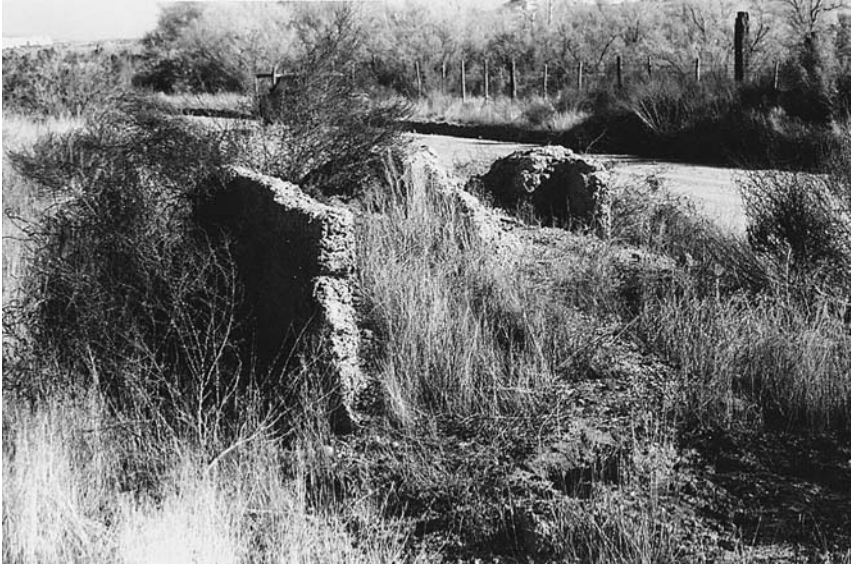
These foundations of houses at Westwater have been destroyed since this photo was taken in 1981. Photo from Wilford Hill files courtesy of Elsa Spaulding Hill.
