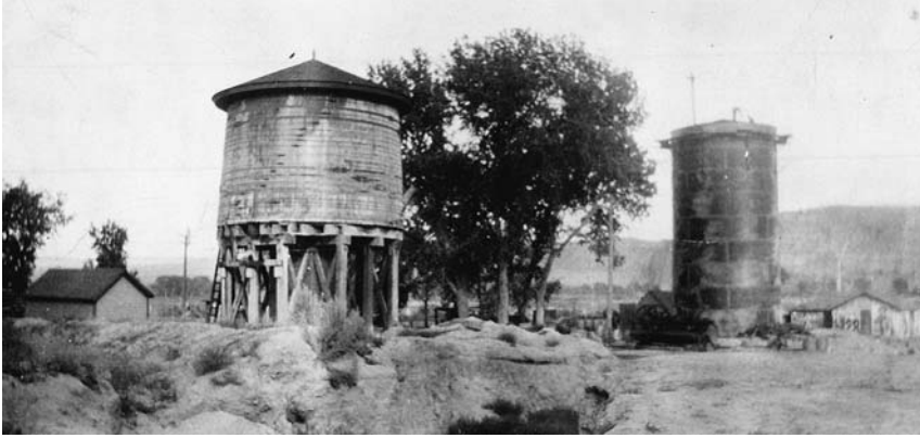
Westwater water tanks. The railroad tank on the left was replaced in 1928. Photo courtesy of Roberta Knutson.
