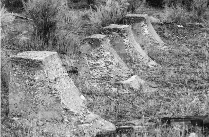
Concrete forms on Westwater Ranch may have once held a 25,000 gallon fuel tank that was needed for a pump W. P. Martin purchased for the ranch in 1916.
