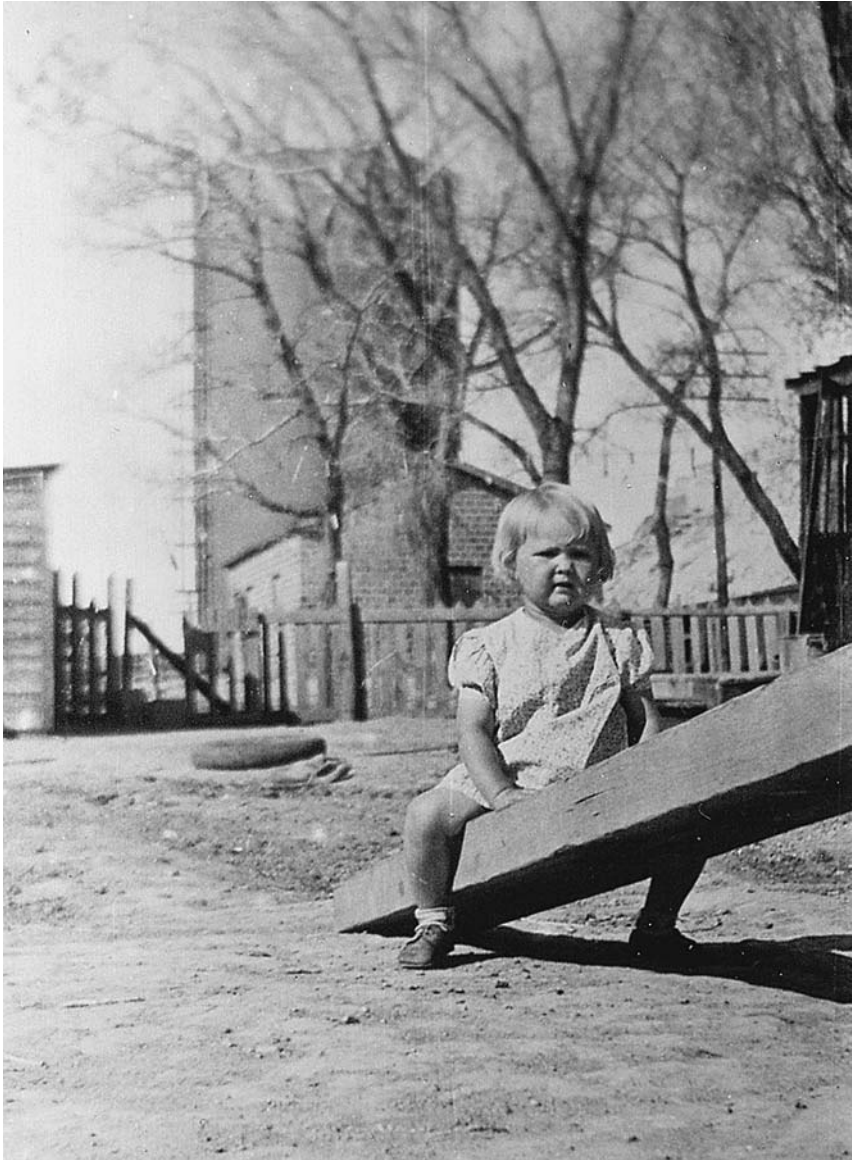
Mickey Thompson, age two, playing in front of the Westwater water tank and the brick treatment plant in 1931. Her father built the merry-go-round/teeter-toter Mickey is playing on. Photo from the Wilford Hill files courtesy of Beryle Marah.
