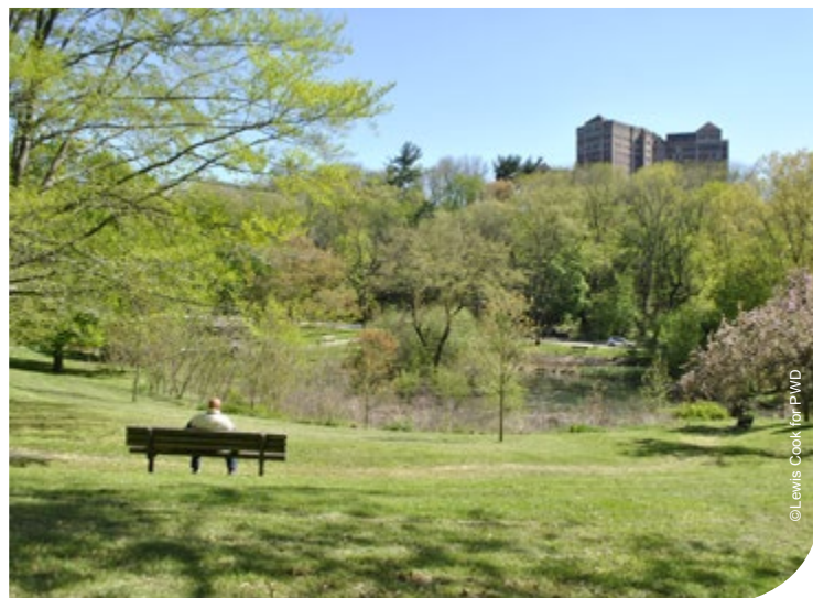
This one-acre stormwater wetland was constructed in Philadelphia to treat stormwater runoff in an effort to improve drinking water quality while minimizing the impacts of storm-related flows on natural ecosystems.
