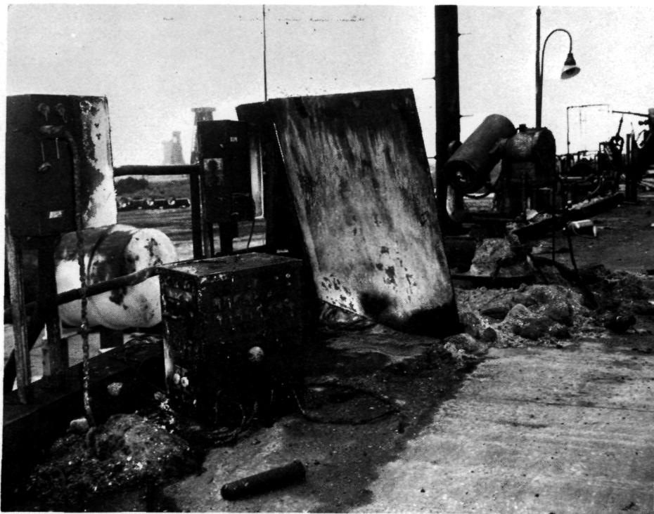
Figure XII-10. - View at top of ramp showing typical destruction of electrical equipment and cameras.
