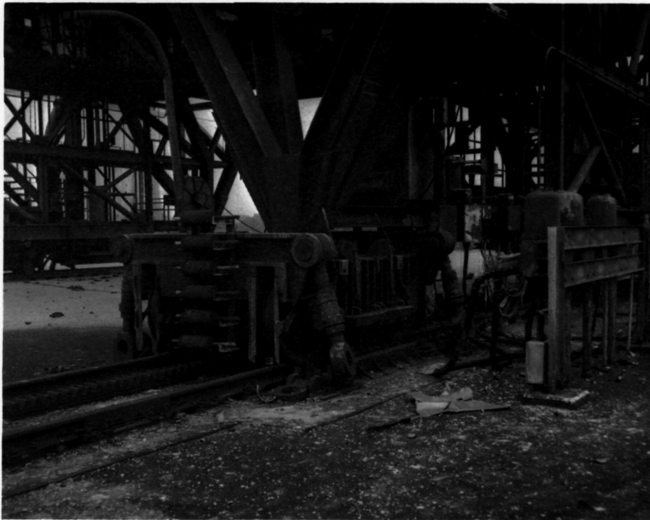
Figure XII-3. - View of southeast corner of service tower showing heat damage to electrical wiring.
