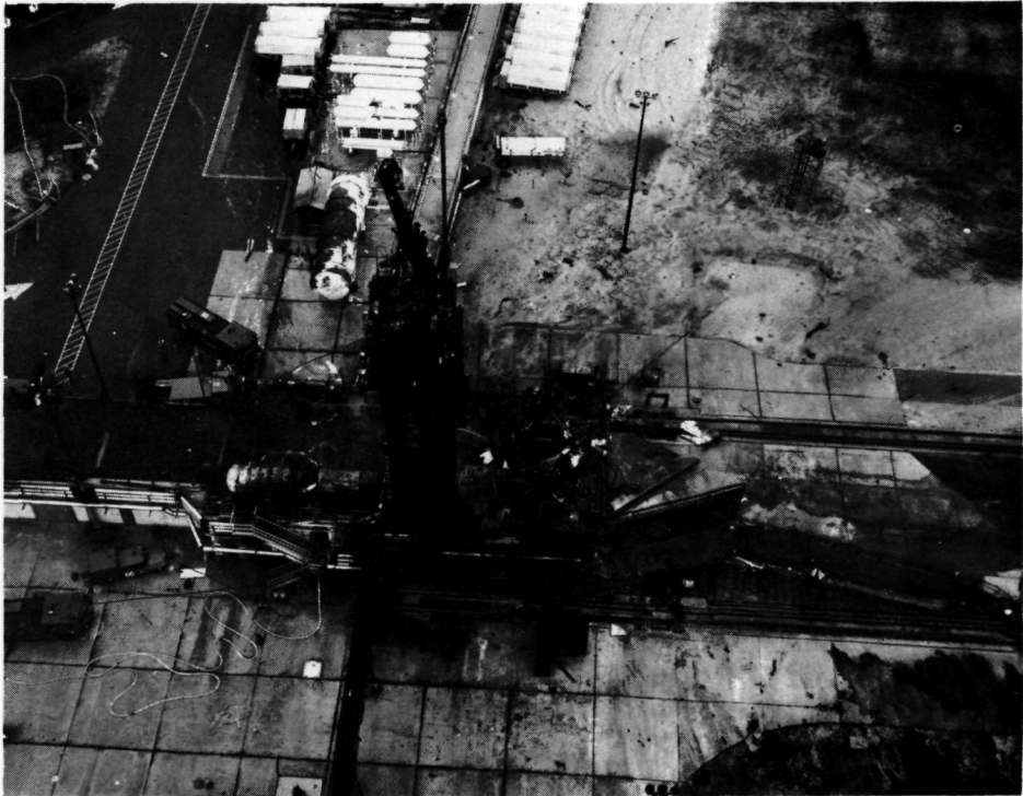
Figure XII-1. - Aerial view showing general damage to pad area.
