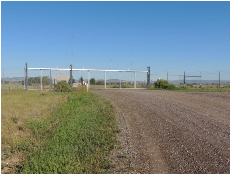
Fig. III.A.15. Motorized entrance gate at WWVB site.
