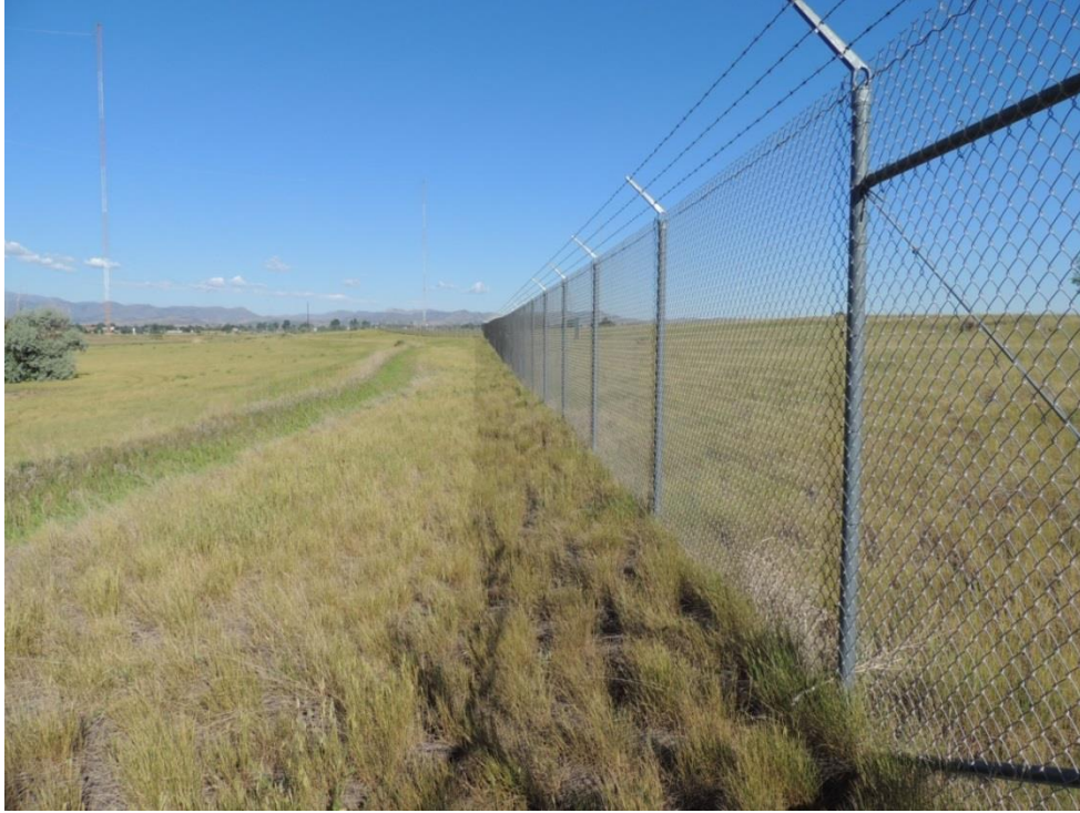
Fig. III.A.16. Portion of perimeter fence at WWVB facility.
