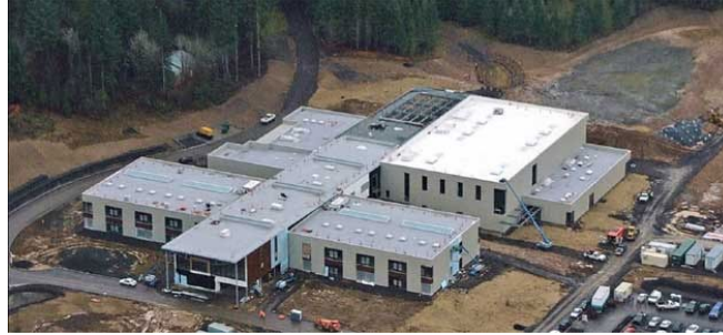
Figure 4-3. Vernonia New Schools Under Construction (source: Oregon Solutions).
