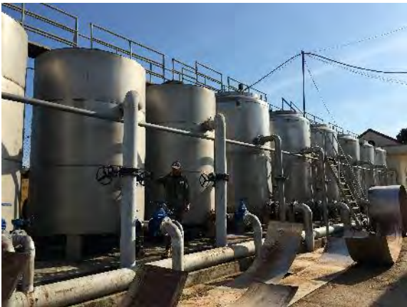
FIGURE 3. DOI SON WATER TREATMENT PLANT
