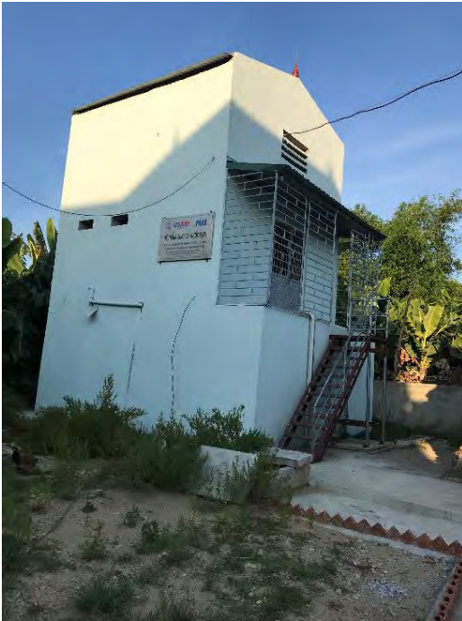
FIGURE I. WATER PLANTS IN CHUE CAU VILLAGE
