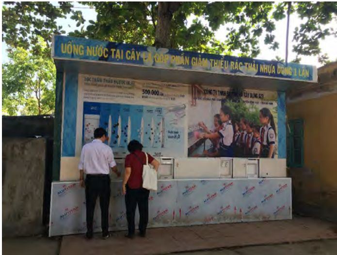
FIGURE 4. WATER PURIFICATION PLANT IN TRANG AN COMMUNE
