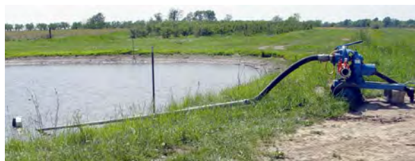
Figure 3-6-A. Portable pump at irrigation pond.
